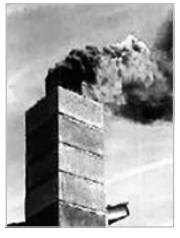
A chimney fire originates in the chimney and is the burning of deposits of soot or creosote
